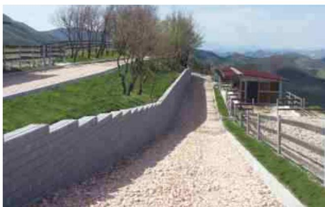
**MURO A SECCO INCLINATO DI 8°**
